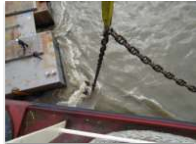
Photo 9: Floating crane barge assistance in recovering an anchor
