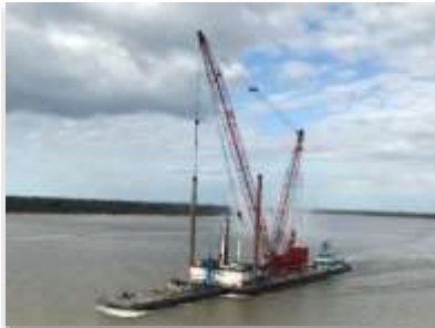
Photo 8: Typical crane and/or deck barge assistance
