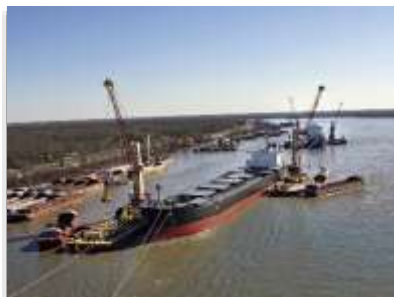
Photo 5: A typical midstream mooring facility (2)
